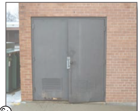
⑥A HOLLOW METAL DOORS & HOLLOW METAL FRAME
